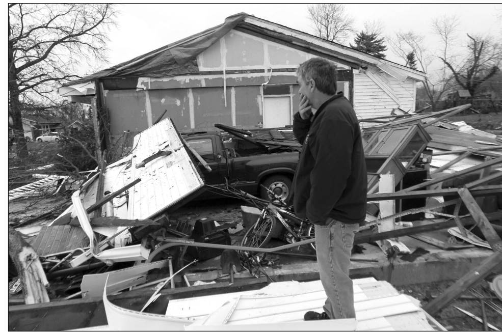
Laurie Skrivani/St. Louis Post-Dispatch/MCT Alan Besaw looks over damage to his garage and truck at his on Townhouse Lane in Hazelwood suburb in St. Louis, on Thursday.
