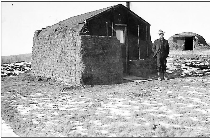
P&D ARCHIVE PHOTO Sod houses like these were common in Yankton's earliest days. "During a long rainy spell, it continued to rain in the house for several days after the skies had cleared outside and mother kept tin pans about the floor to catch the drips," recalled one pioneer.
