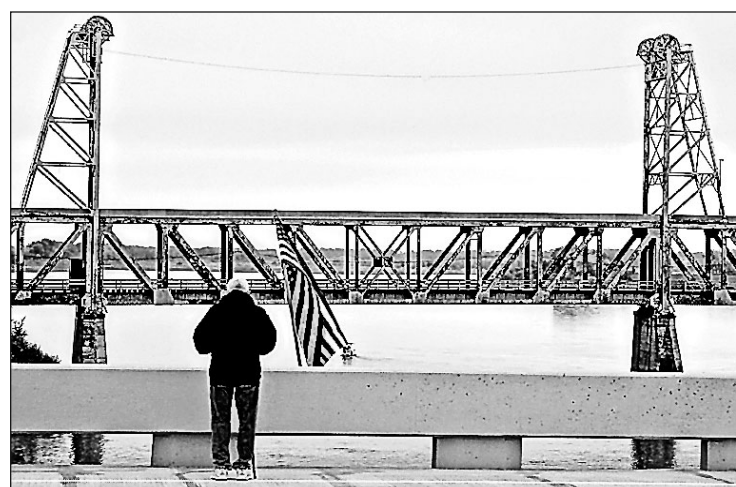
An individual looks over at Meridian Bridge from its replacement, the Discovery Bridge, during the opening ceremonies for the new bridge in October 2008.
