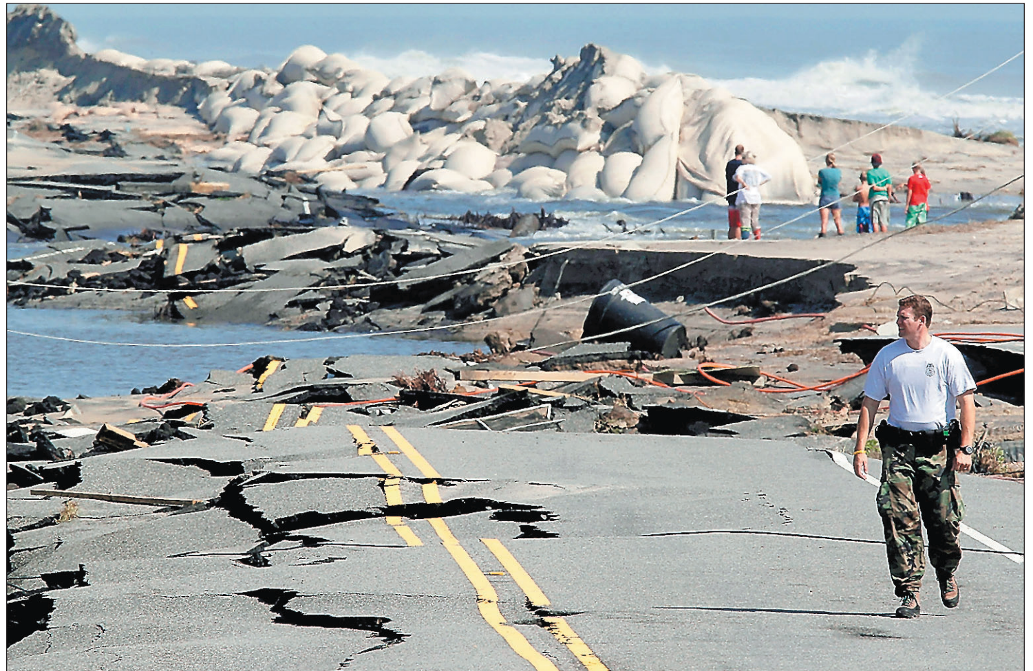
National Park Service Ranger Jeff Goad views the destruction to North Carolina Highway 12 on the north edge of Rodanthe, N.C., Sunday due to the storm surge from Hurricane Irene.
