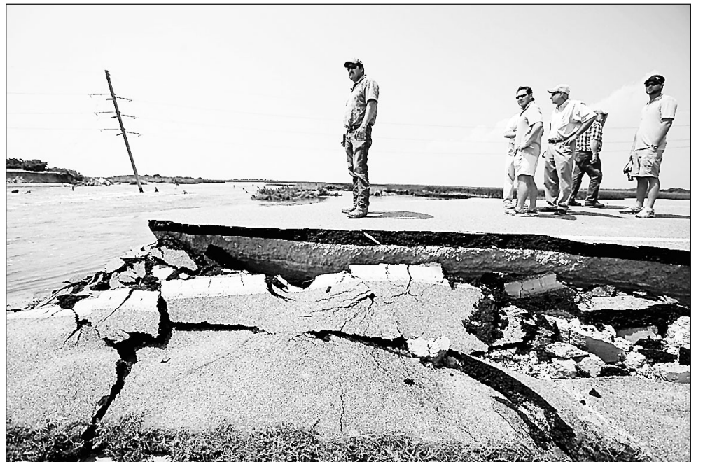
SHAWN ROCCO/RALEIGH NEWS & OBSERVER/MCT Randy Boyd, left, of the North Carolina Department of Transportation, stands on a portion of N.C. 12 that was washed away near the Pea Island National Wildlife Refuge in North Carolina on Monday. He and three other DOT officials and a contract survey crew came down to assess the damage caused by Hurricane Irene.
