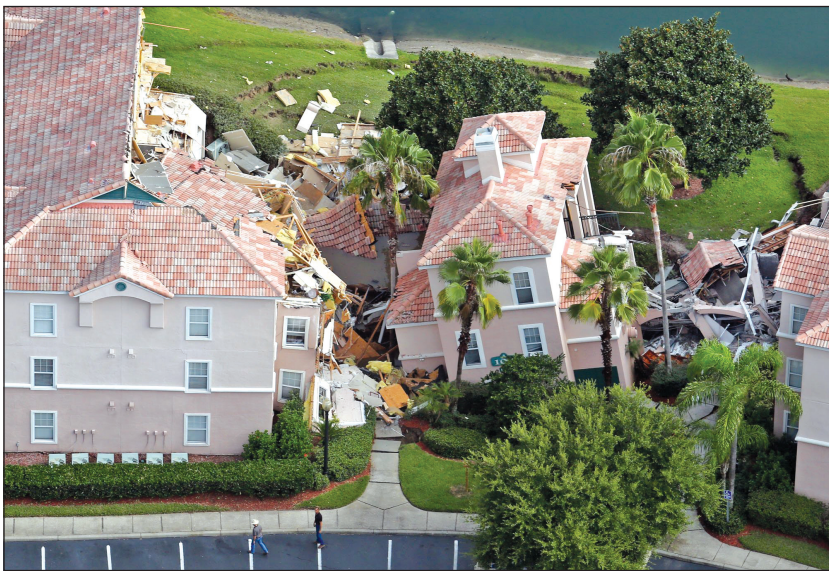
RED HUBER/ORLANDO SENTINEL/MCT Guests had only 10 to 15 minutes Monday to escape the collapsing buildings at the Summer Bay Resort on U.S. Highway 192 in the Four Corners area, located about 7 miles east of Walt Disney World resort, where a large sinkhole — about 60 feet in diameter and 15 feet deep — opened in the earth late Sunday.
