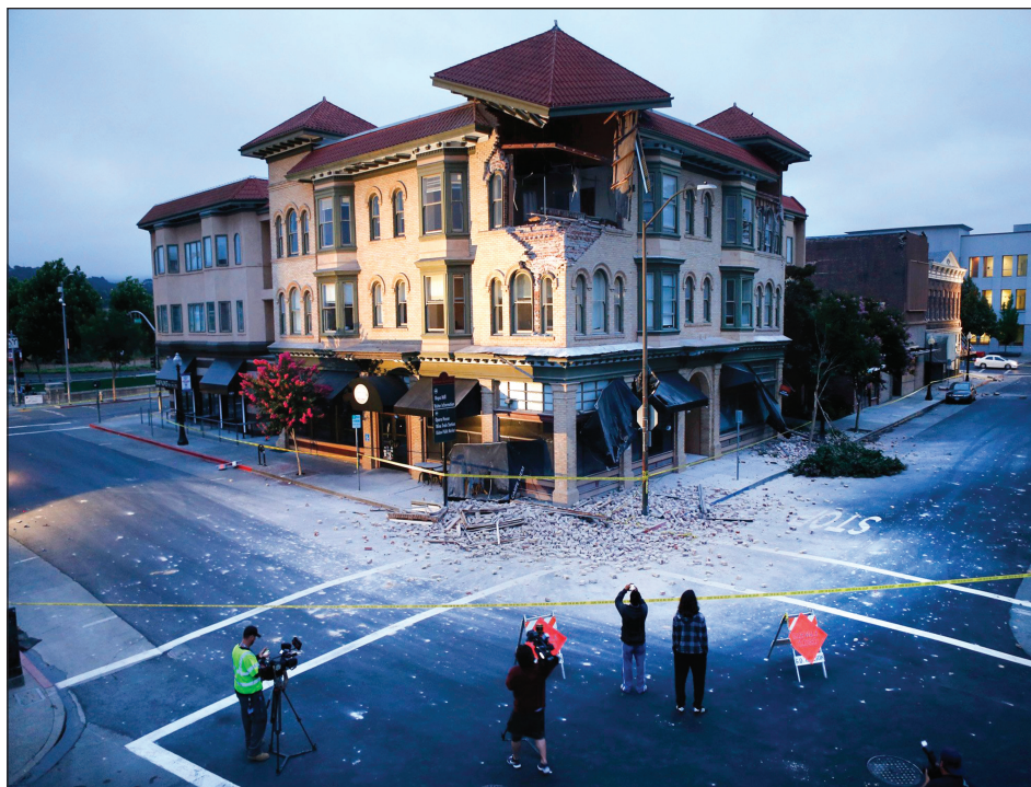
The Alexandria Building in downtown Napa, Calif., was severely damaged by the 6.0 earthquake that struck the Bay Area on Sunday.
