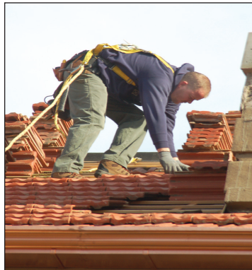
DAKOTA TERRITORIAL MUSEUM A worker from Stonebrook Roofing is shown installing clay tiles on top of the Mead Building in Yankton earlier this week. The roofing project is part of the ongoing effort by the Yankton County Historical Society to renovate the historic building.
