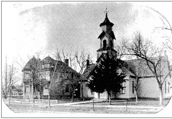
Old Parish House 601 Maple Street
