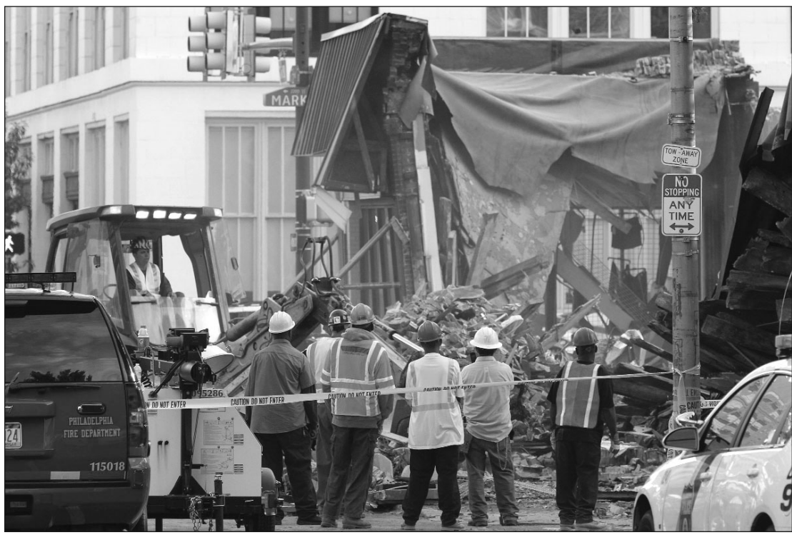
ALEJANDRO A. ALVAREZ/PHILADELPHIA DAILY NEWS/MCT Demolition crews stand behind the Salvation Army store to start working Thursday in Philadelphia, Pennsylvania. A downtown Philadelphia building that was undergoing demolition toppled onto a busy Salvation Army thrift shop Wednesday, killing at least six people and injuring 14, the last of whom was pulled from the debris just before midnight.
