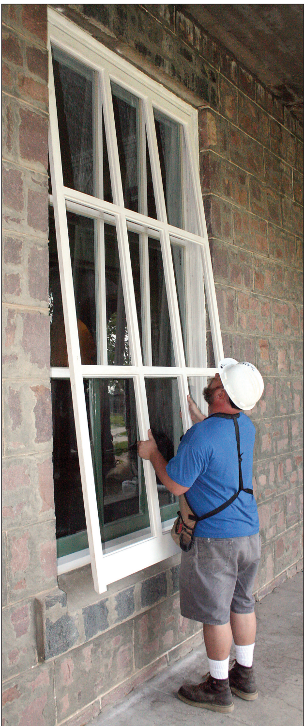
Ben Brunick of Chalkstone Woodworking demonstrates one of the new storm windows that are being built and installed at the Mead Building ROB NIELSEN/P&D
