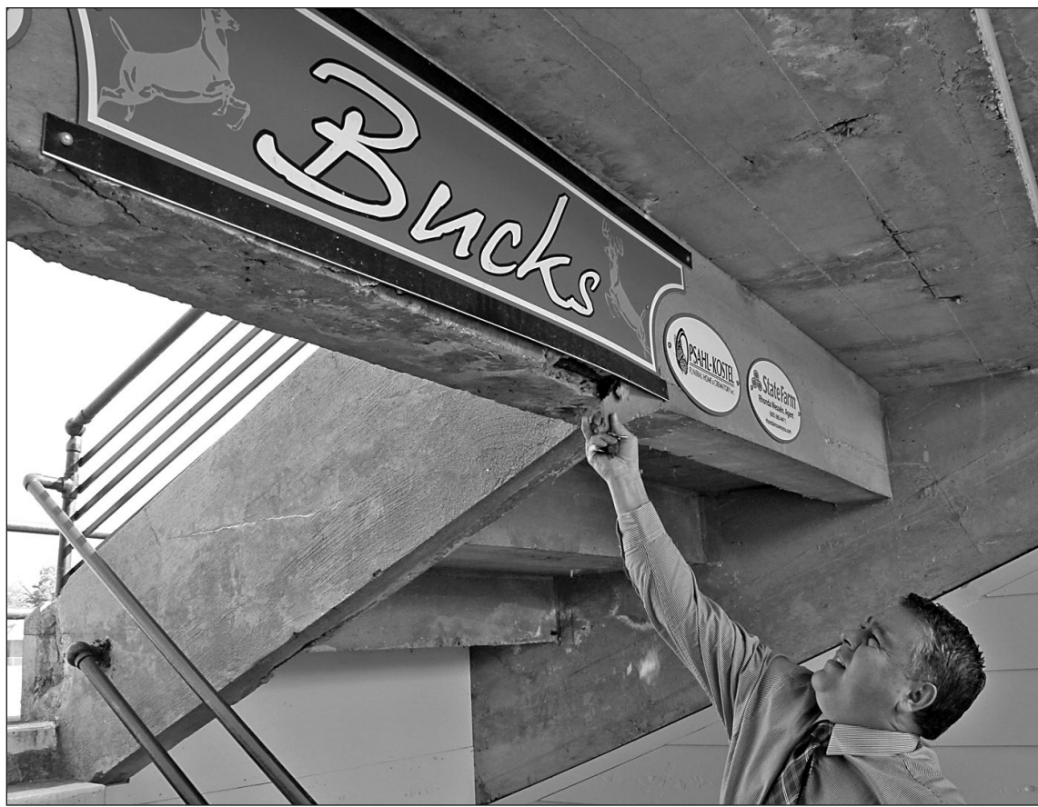
Yankton School District Superintendent Dr. Wayne Kindle pointed to this crack near a sign during a tour of Crane-Youngworth Field Friday — and a small chunk of concrete fell off debris fell out. Wiring issues and inadequate facilities are also problems faced at the facility.
