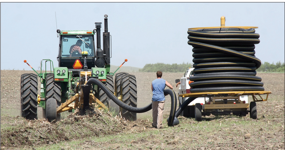
KELLY HERTZ/P&D A crew from Kokes Ag Service of Tabor begins work inserting tiling into a cornfield east of Utica Friday. The Yankton County Commission has instituted a drainage ordinance that was drawn up in part to the growing popularity of tiling among farmers.
