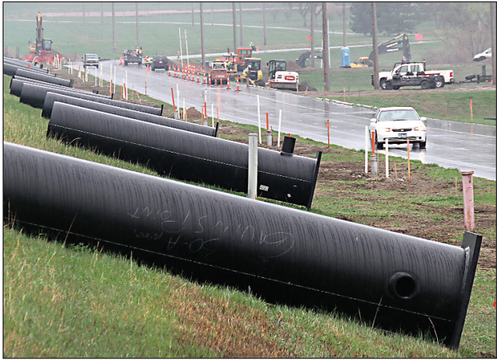
These large tubes have been lining Toe Road below Gavins Point Dam recently. These tubes, which are 10 feet long and three feet in diameter, are manholes for relief wells that are being installed along the dam. The tubes will allow inspectors access to the wells. It is part of an approximately $20 million package of upgrade in the dam area.
