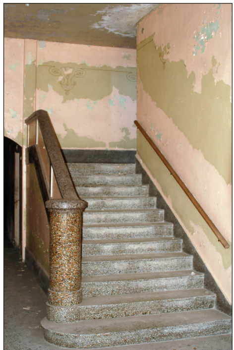
PHOTO: DAKOTA TERRITORIAL MUSEUM This interior shot of a staircase leading to the second floor on the Mead Building also shows some of the paint that is peeling off the walls. Also visible is the stenciling that has been documented as part of the restoration project.
