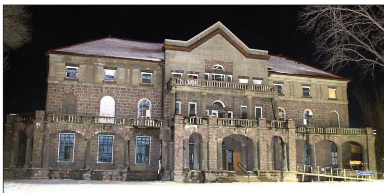
KELLY HERTZ/P&D The Mead Building restoration project will host a fundraiser this weekend, as members of the public can reserve blocks of time to have photos taken on the building's marble staircase.
