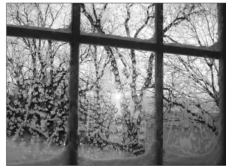
PHOTOS COURTESY OF METROCREATIVE SERVICES Warm, moist interior air meeting up with cold air from outside can cause window sweating.
