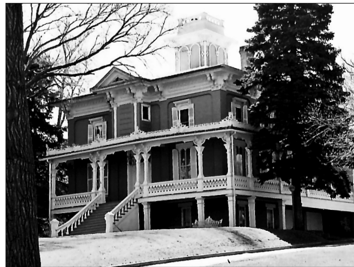
THE SHANNON-OHLMAN HOUSE Built By Peter C. Shannon (1874) 205 Green Street
