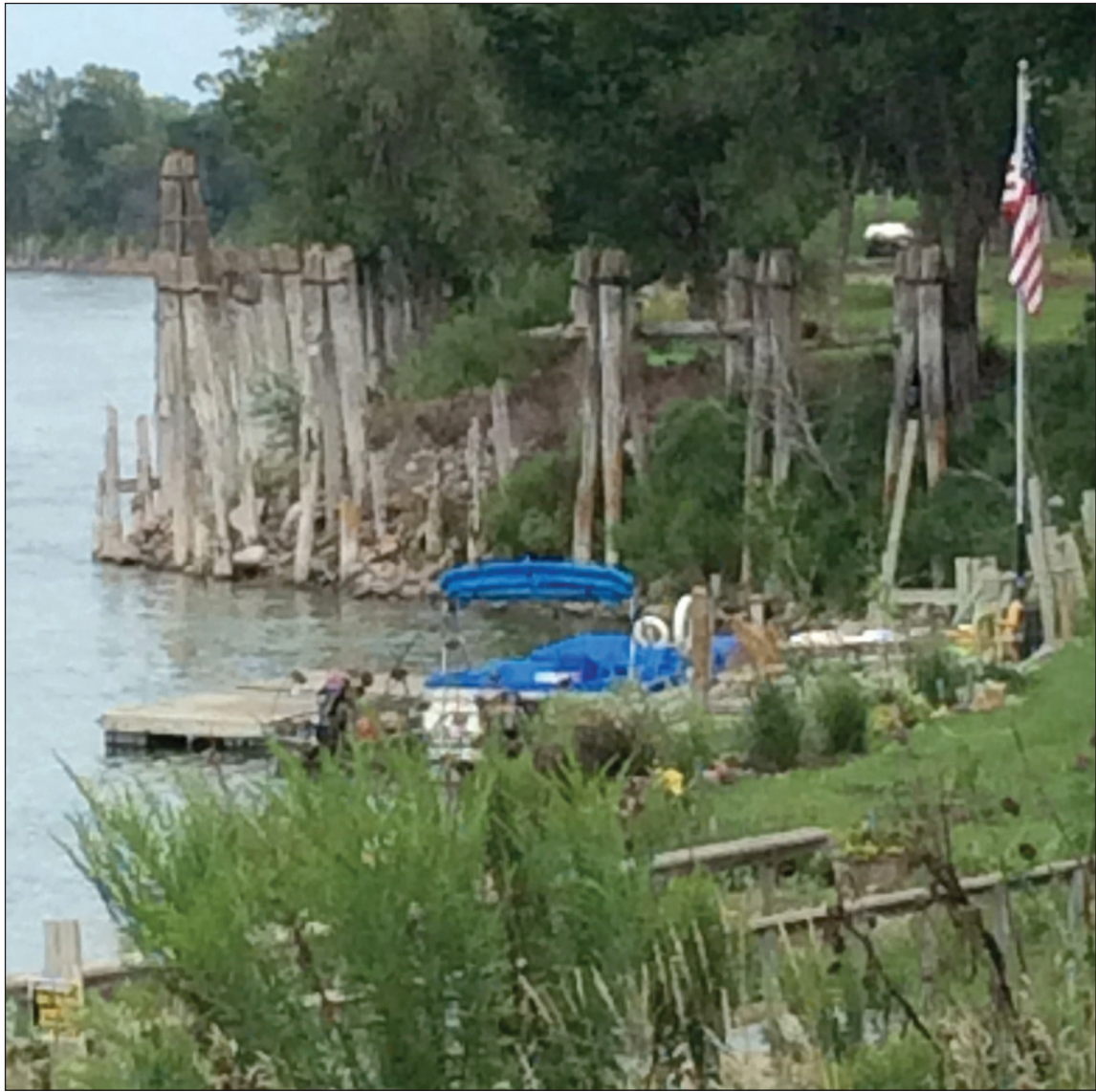
These pilings located along the south side of the Missouri River west of Yankton are remnants of the bank fortification work done by German prisoners of war who were assigned here late in World War II.
